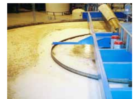
Sand filtration treatment of effluent water
