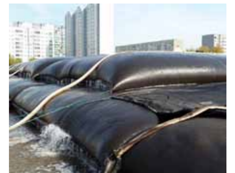
Dewatering two layers of Geotube ® containers
