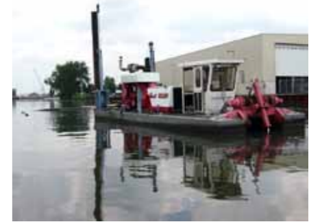
Dredging of contaminated sediment*
