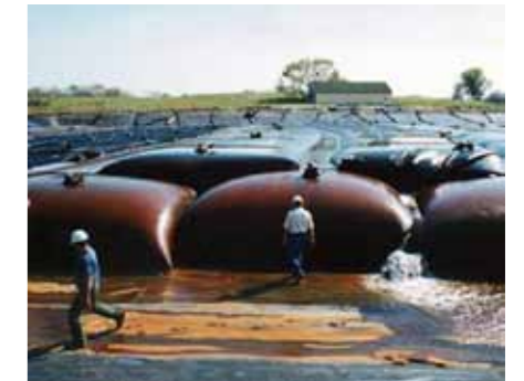
Geotube ® dewatering containers within the containment facility
