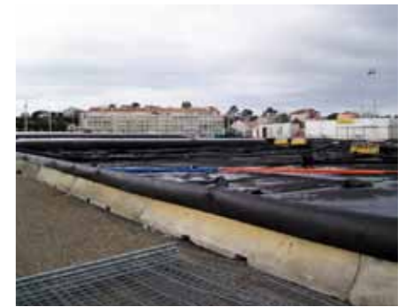
Geotube® dewatering cell laid out on East breakwater
