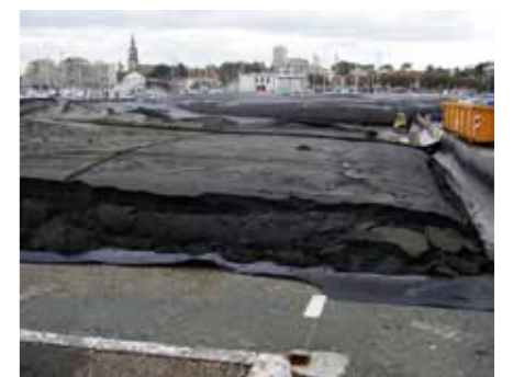
Dewatered contaminated sediment ready for offsite disposal
