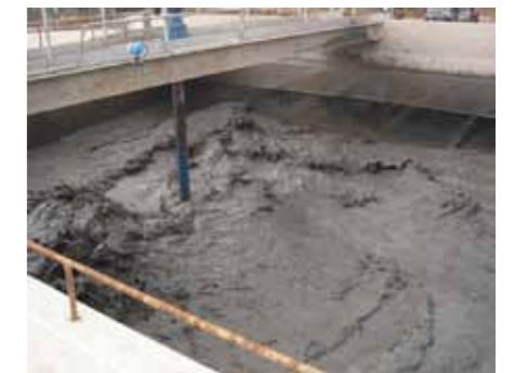
Agitation of slurry fines in a holding tank
