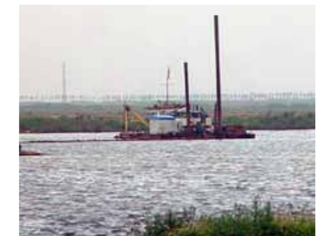
Dredging contaminated sediments from the impoundment lake
