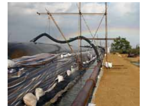
Filling Geotube® containers with contaminated sediments
