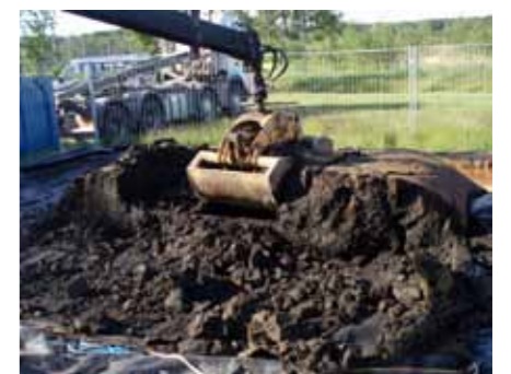
Excavation of dewatered solids for transport to offsite disposal facility
