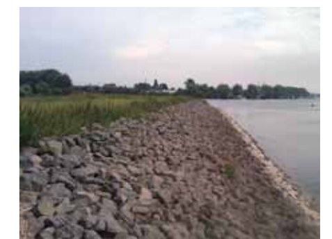
Completed riverbank restoration
