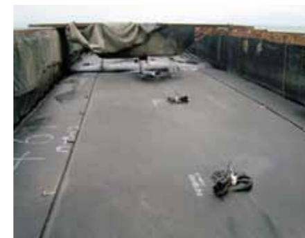
Offshore Geotube® contained disposal of contaminated sediments
