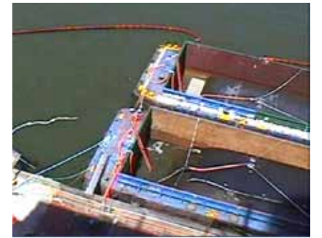
Geotube® dewatering containers in barges in East River
