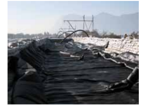
Installing Geotube® containers inside the geobag buttress walls
