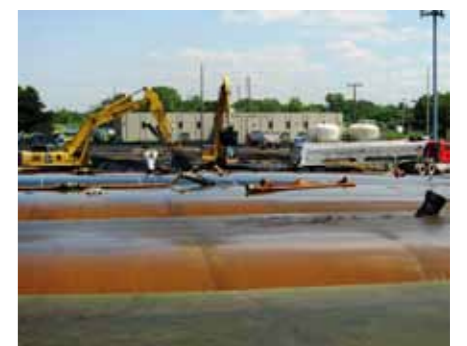
Final dewatering and transport of dewatered contaminated sediment to offsite disposal facility
