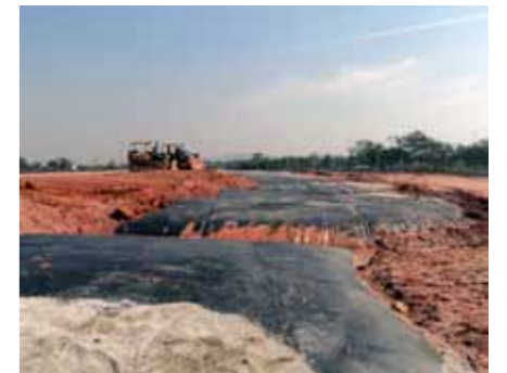
Capping a Geotube ® dewatering cell
