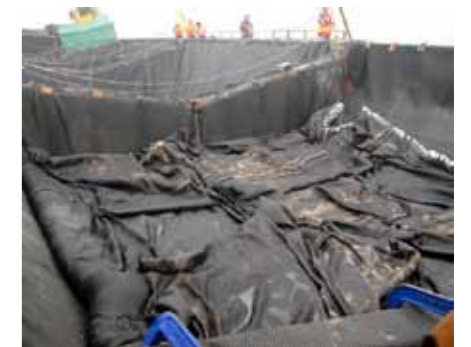
Filled Geotube® container dropped through split-bottom barge at offshore dumpsite
