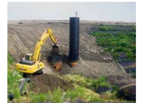
Earthfill levelling course over dewatered Geotube® containers
