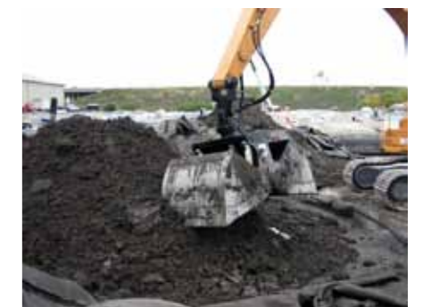
Removal of dewatered contaminated sediment to external landfill
