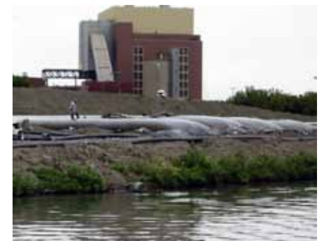
First layer of Geotube ® containers filling with dredged contaminated sediments
