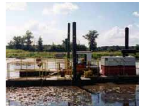
Dredging contaminated sediment in West Branch Grand Calumet River
