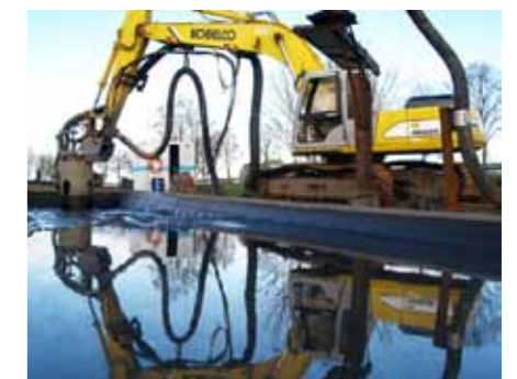
Pumping slurry from docked transport barge to Geotube ® dewatering platform
