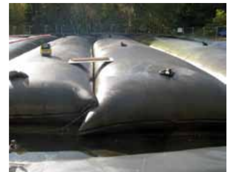
First layer of Geotube ® dewatering containers filled
