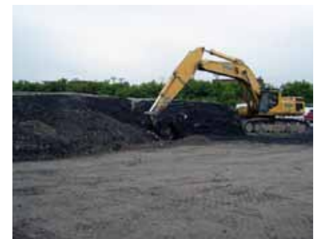
Excavation of dewatered sediment for transport to offsite disposal facility
