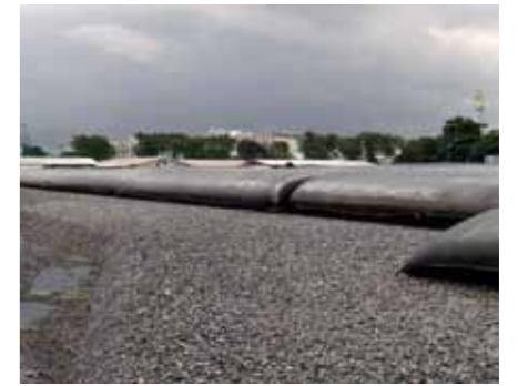
Geotube ® dewatering platform
