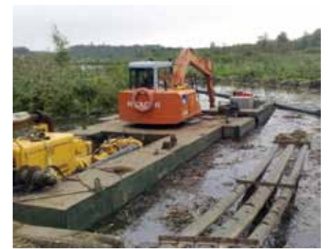
Dredging of contaminated sediments in Sorte Sø
