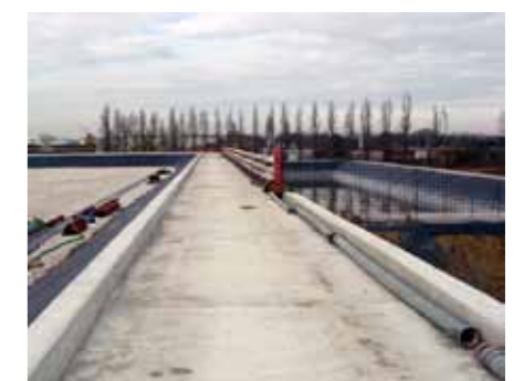
Water effluent pond adjacent to dewatering facility
