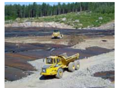
Capping of the dewatering platform
