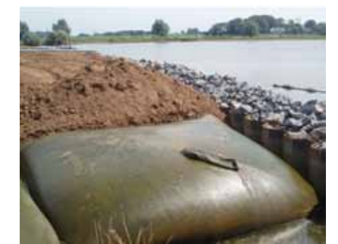
Placing earthfill covering over dewatered sediments
