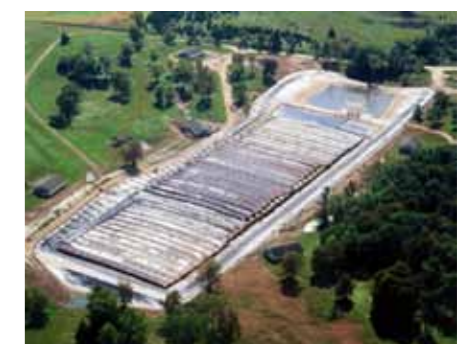
Overview of the Geotube ® dewatering facility
