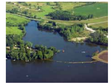
Dredging of Grubers Grove Bay
