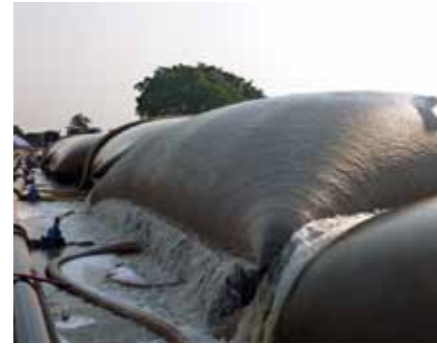
Geotube® technology used for environmental engineering
