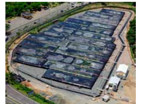
One of the Geotube ® dewatering cells
