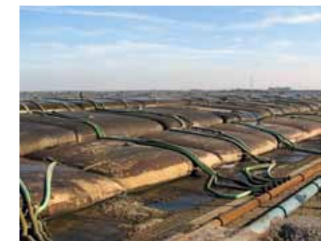
Three layers of Geotube ® containers on the dewatering platform
