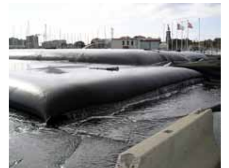
Dewatering contaminated sediment
