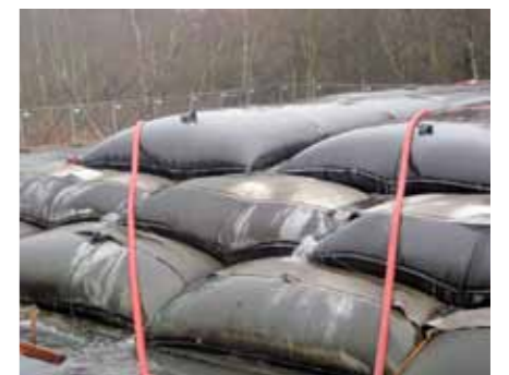
Geotube ® dewatering containers stacked three high
