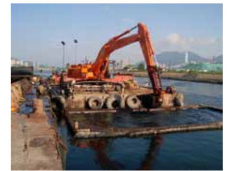
Mechanical dredging of contaminated sediments at Kai Tak
