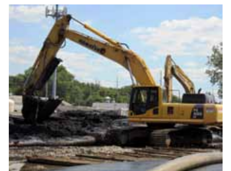
Excavation of dewatered contaminated sediment for offsite disposal
