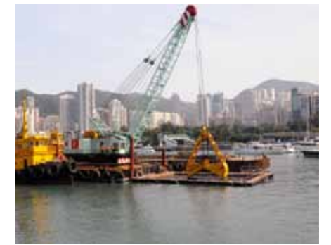
Dredging contaminated sediments at Wan Chai
