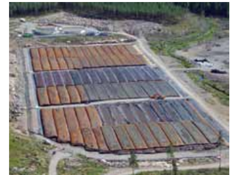
Geotube ® dewatering platform with the water treatment plant shown on the far side
