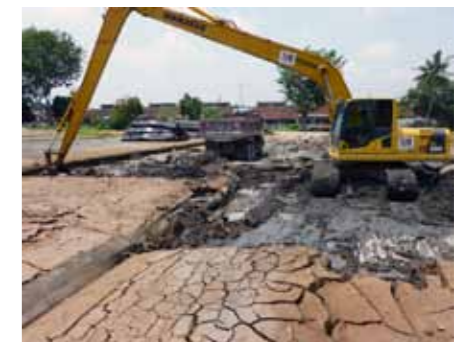
Excavation of dewatered contaminated sediments for transport to offsite landfill
