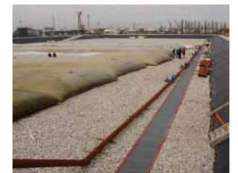
Filled Geotube ® units in the constructed dewatering platform
