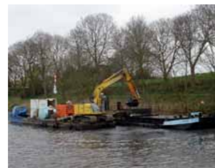
Dredging of contaminated sediment into transport barge
