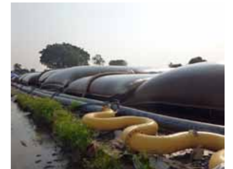
Geotube ® dewatering of contaminated sediments showing slurry delivery pipes
