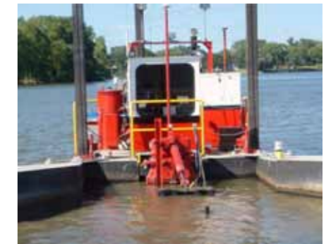
Small scale hydraulic dredge
