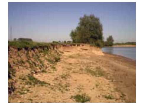
Riverbank erosion on IJssel River at Zutphen
