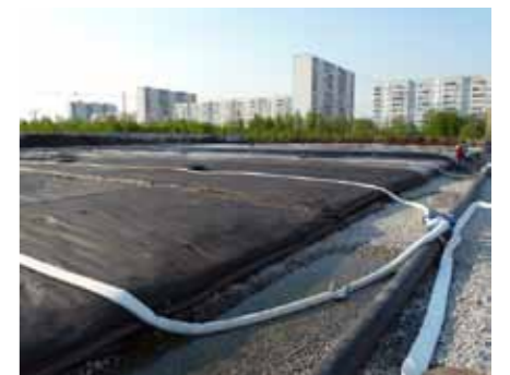
Filling first layer of Geotube ® dewatering containers
