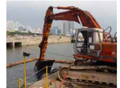
Mechanical dredging using an excavator
