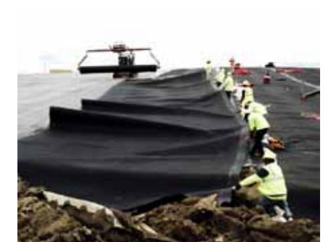
Geomembrane liner installed in cap over Geotube® dewatering facility
