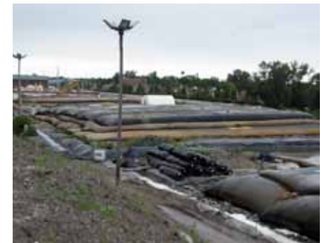
Geotube ® containers stacked three high on dewatering platform
