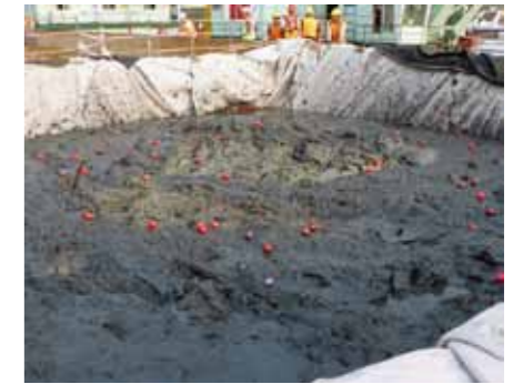
Contaminated sediment placed inside Geotube® container
