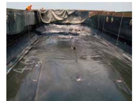
Geotube ® container being dropped through split-bottom barge at offshore dump site
