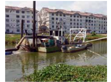
Dredging of contaminated sediments from Melaka River
