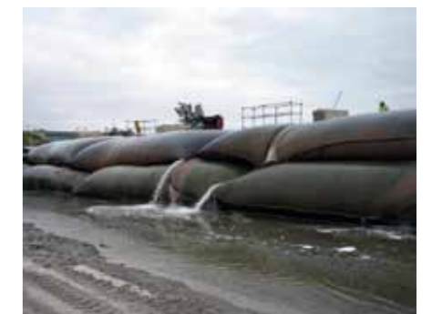
Geotube ® dewatering of contaminated sediments
