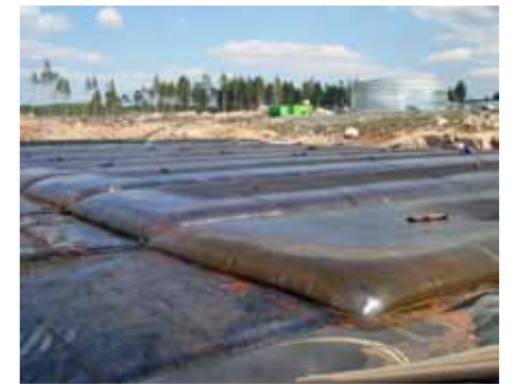
Geotube ® dewatering of the contaminated sediments
