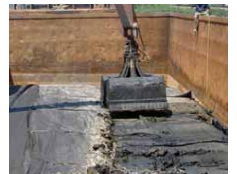
Dewatered contaminated sediment being removed from barge
