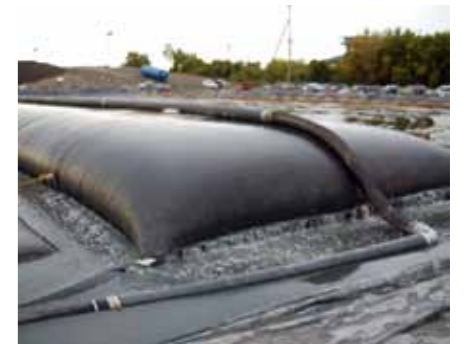
Geotube ® dewatering of contaminated sediment slurry
