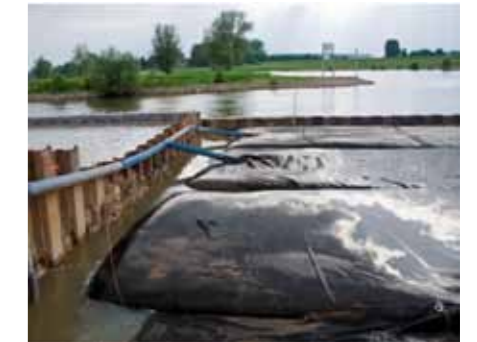
Filling Geotube ® containers with sediment slurry
