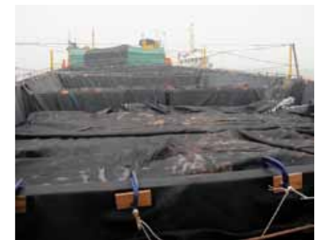
Filled Geotube® container closed and transported to offshore dumpsite
