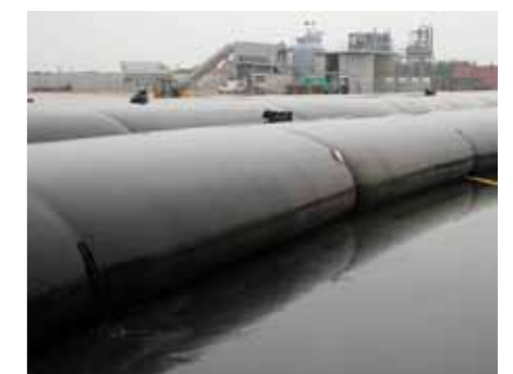
Geotube ® dewatering of contaminated sediment
