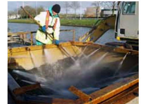
Steel grating used to separate out unidentified explosive objects from contaminated sediment
