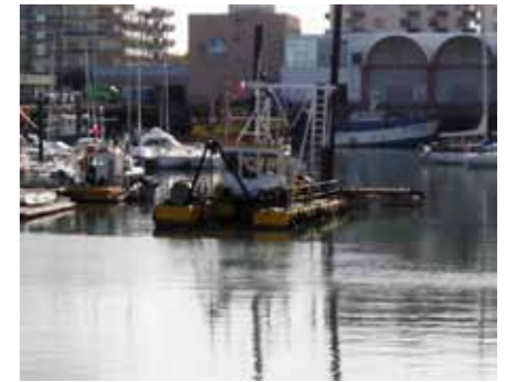
Dredging contaminated sediment in the marina basin
