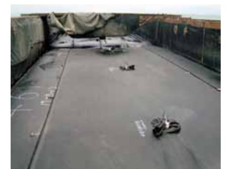
Filled Geotube ® container being taken to offshore dump site
