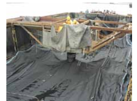
Geotube ® container placed in split-bottom barge
