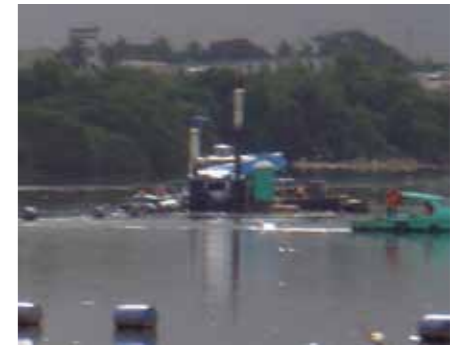
Dredging contaminated sediments in Canal do Fundão
