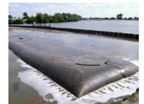
Geotube ® dewatering of sediments
