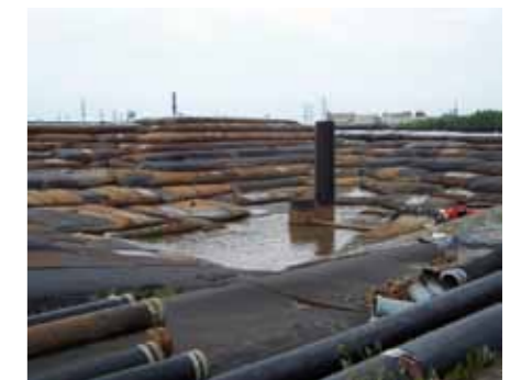
Geotube® dewatering containers stacked 10 high
