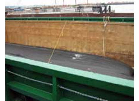
Geotube® dewatering of contaminated sediment in barges
