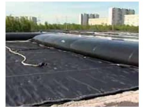
Laying out Geotube ® dewatering containers on dewatering platform
