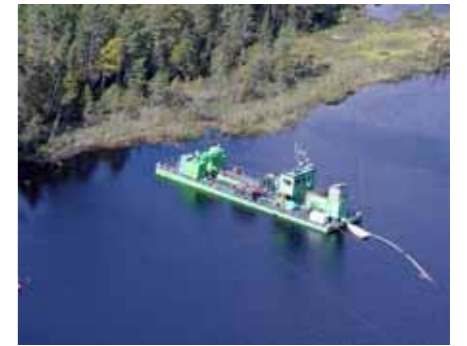
Dredging the contaminated sediments from the lake
