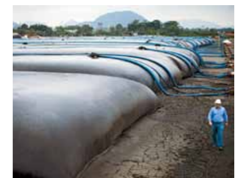
Geotube ® dewatering of contaminated sediments within the earthfill platform
