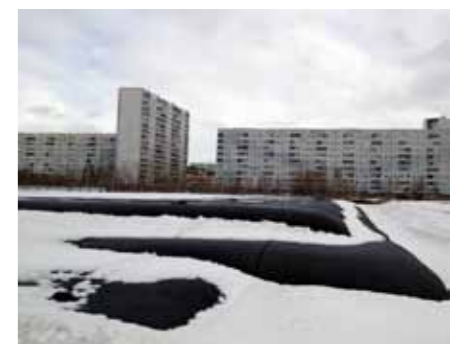
Geotube ® dewatering containers left in place during Siberian Winter
