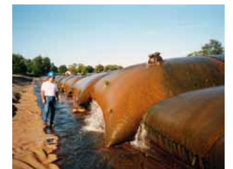
Geotube ® dewatering of the contaminated sediments
