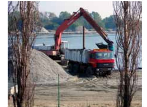
Loading contaminated sediments into a truck for transport to washing plant
