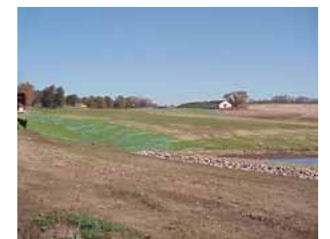
Dewatering facility capped and grassed
