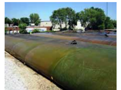
Geotube ® dewatering platform
