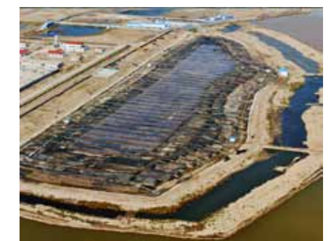
Geotube ® dewatering platform
