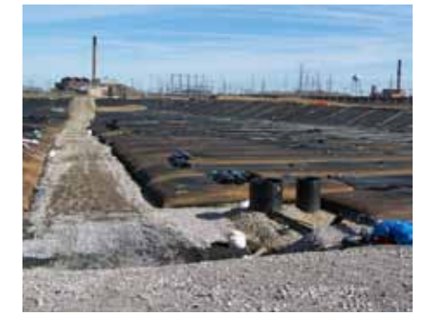
First layer of Geotube® containers in dewatering facility
