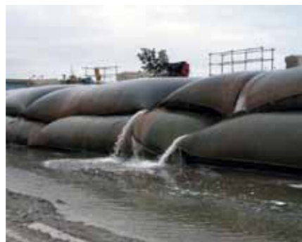
Onshore Geotube® dewatering of contaminated sediments
