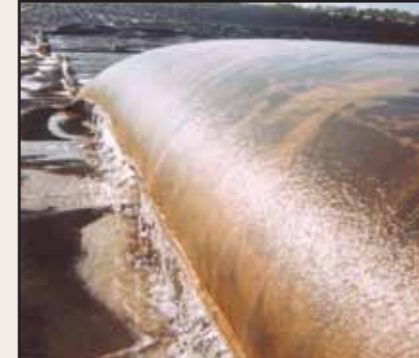
Water draining from a Geotube® container.
