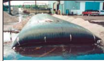
Coal sludge dewatering using Geotube® dewatering technology
